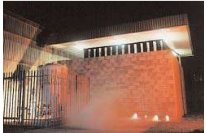
Cryogenic Test Facility/Explosion Proof Chamber.
